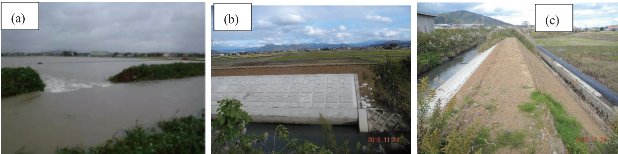
Fig.14 (a) Breach of Jinzuu river (Oct. 23, 2017) (4) , and (b),(c) the restored embankment of Jinzuu river (Nov. 24, 2018).
