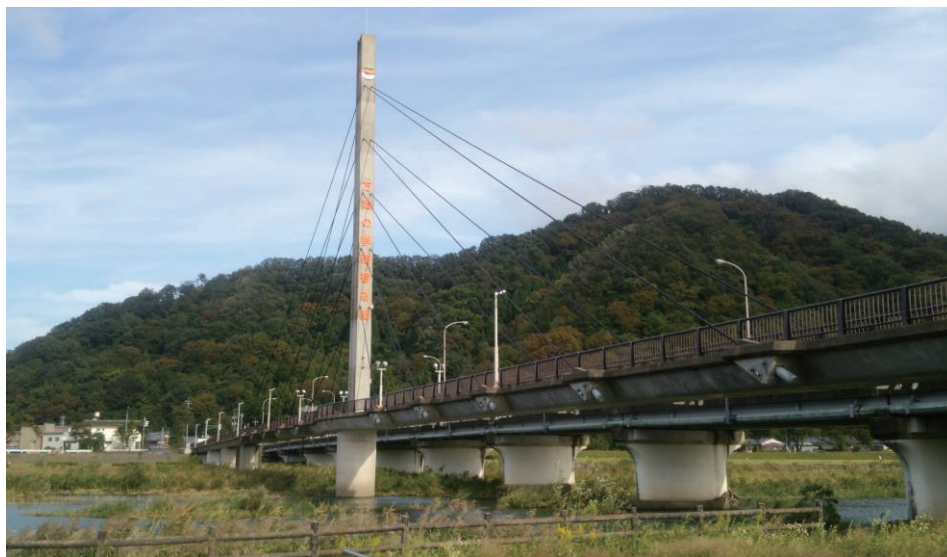
Fig.2 Photo of the overview of Bandai cable-stayed bridge constructed in 1991
