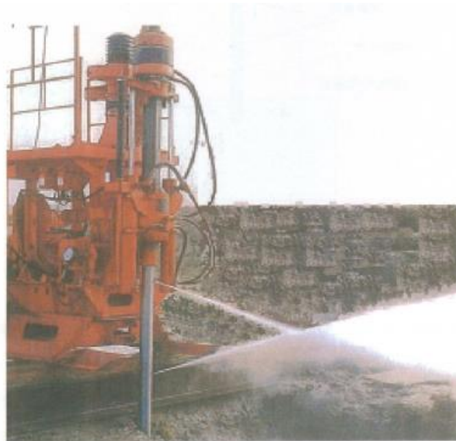
Fig.3. 1 Photograph of High-Speed Water Jet Utilized Soil Improvement
