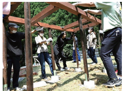
Fig.12 Installing columns and beams
