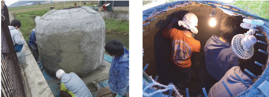
Fig. 3 Lamination work of mortar for the pumpkin tank production.
