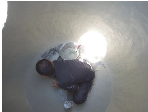
Fig. 4 Waterproofing work for inside of the pumpkin tank.
