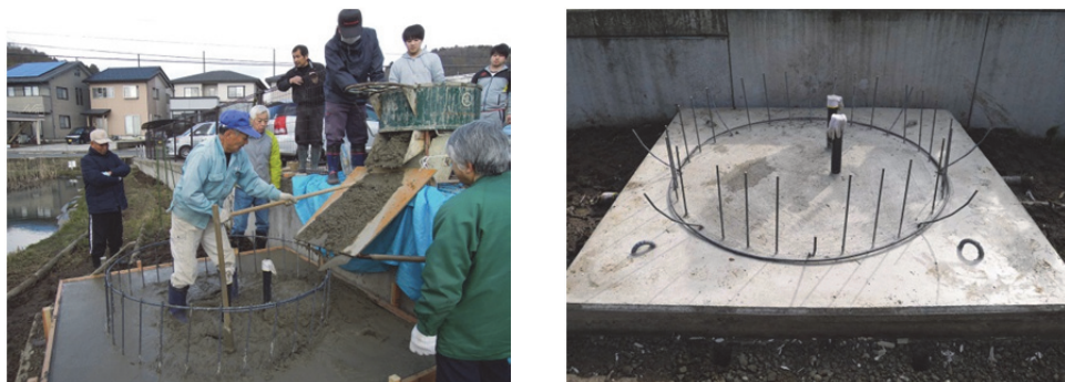
Fig. 2 Foundation work of the pumpkin tank.
