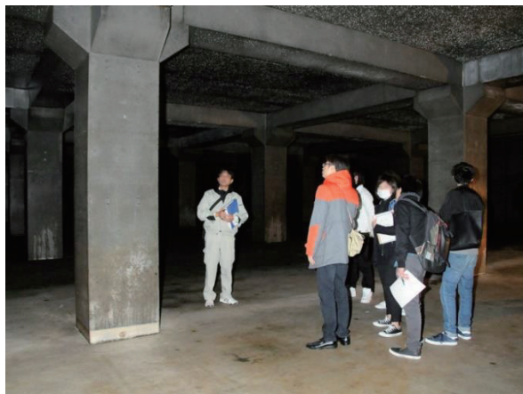
Fig. 2 The inside of the rainwater storage tank of MAZDA Zoom-Zoom Stadium Hiroshima.
