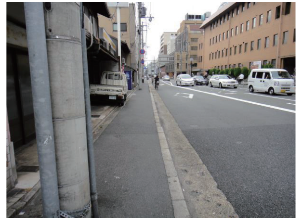
Fig.6 The road status of the surrounding survey area (North)
