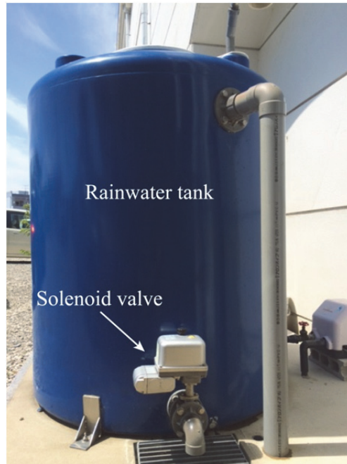
Fig. 5 Rainwater tank with a solenoid valve
