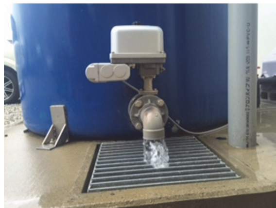
Fig. 10 Drainage from rainwater storage tank
