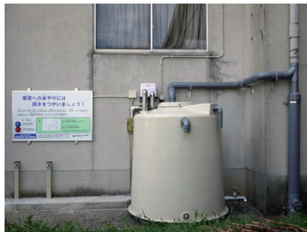
Photo 1 Rainwater catchment system installed in an elementary school
